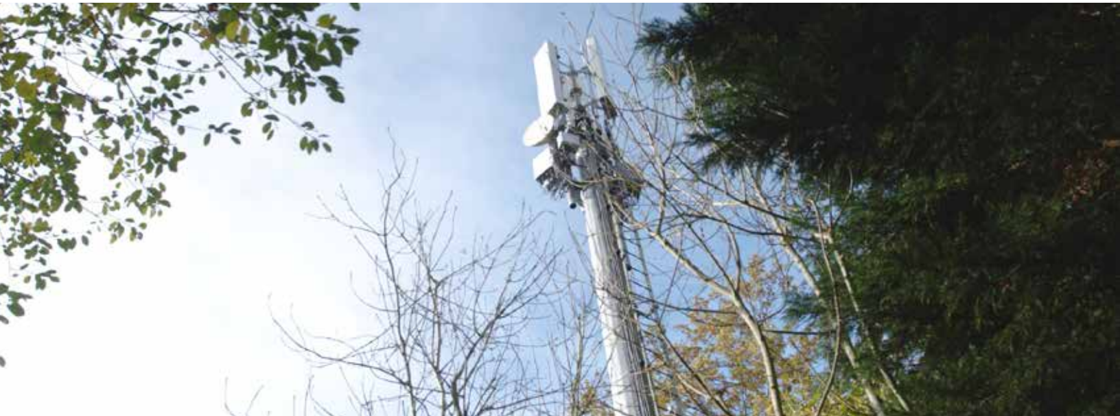
Vodafone UK's first 5G Open RAN site
